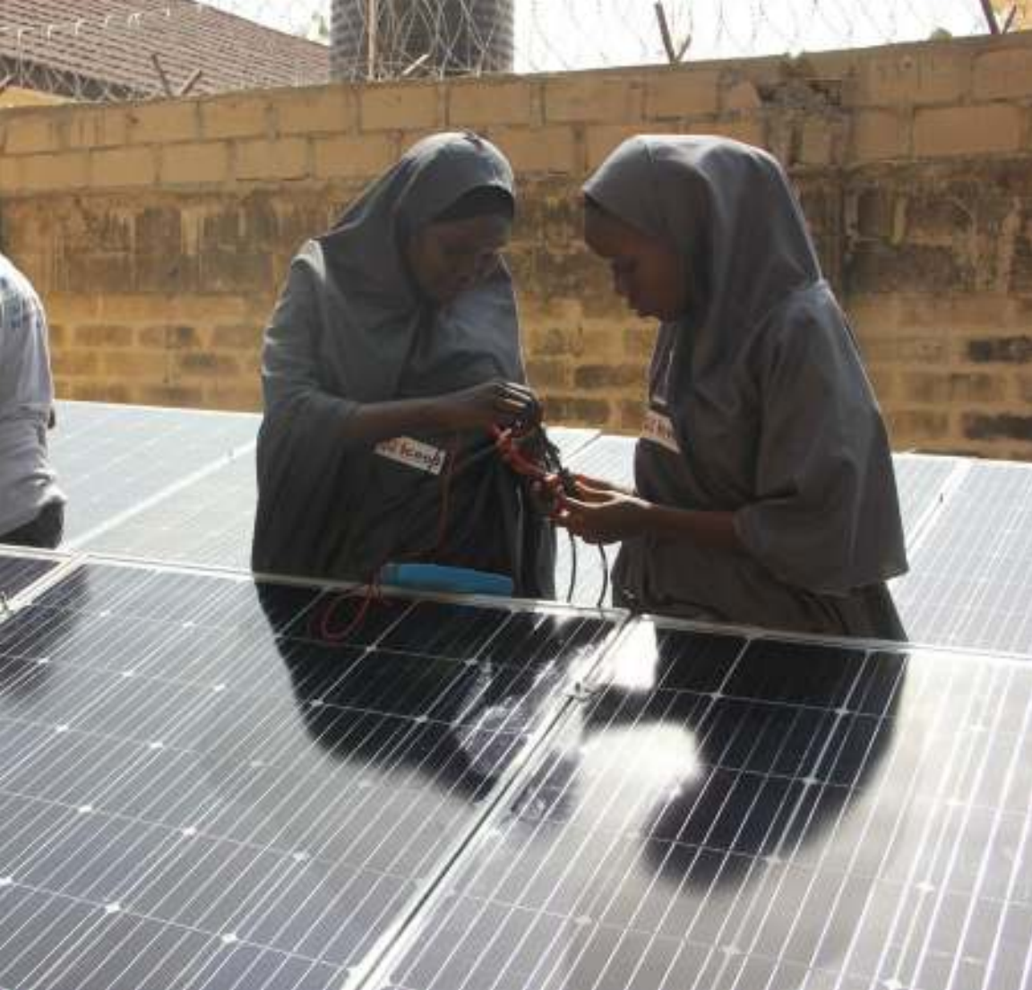
Solar technician training
