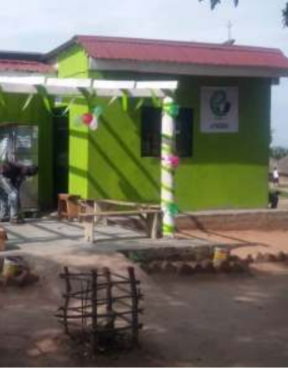
Energy Kiosk in Rhino Camp Refugee Settlement
